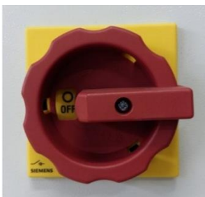
Main switch OFF
