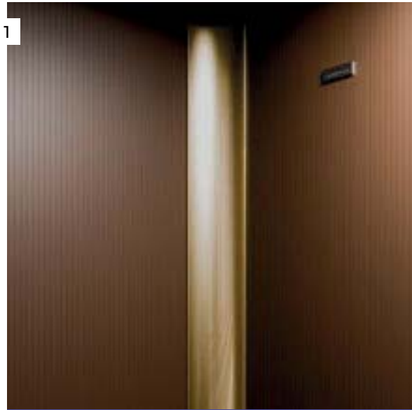
1- Column and wall in anodised aluminium.
